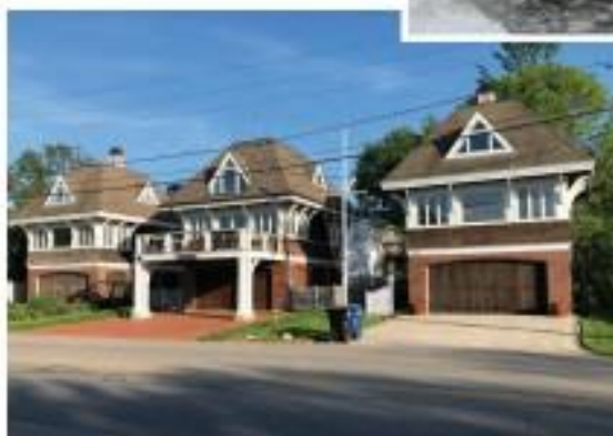
Three single-family homes farther west on Wellington were elevated when built in 1988. According to Newport Building Official, William Hanley, FEMA's base flood elevation in this area is 13 ft. That's 1 ft. higher than in the point because it is a Velocity Zone where wave action of 1 1/2 ft. can be expected from storm surges. In addition to having the first floor elevated higher, the side walls and doors of the garages must break away with any storm surge, leaving the home perched on the upright supports, but otherwise relatively unharmed.
