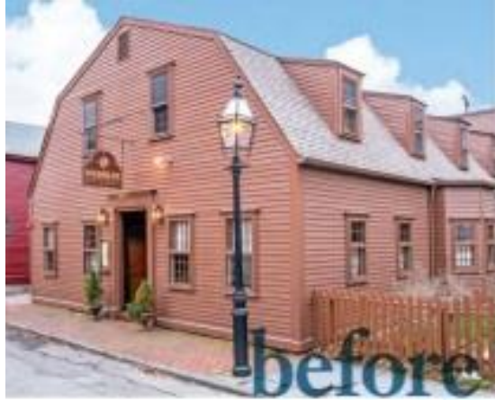
Left: There was only a small, damp crawlspace beneath the Rumble Restaurant at 62-64 Bridge Street when it was listed for sale in 2015. PHOTO: GREGORY ANASTASIAN
